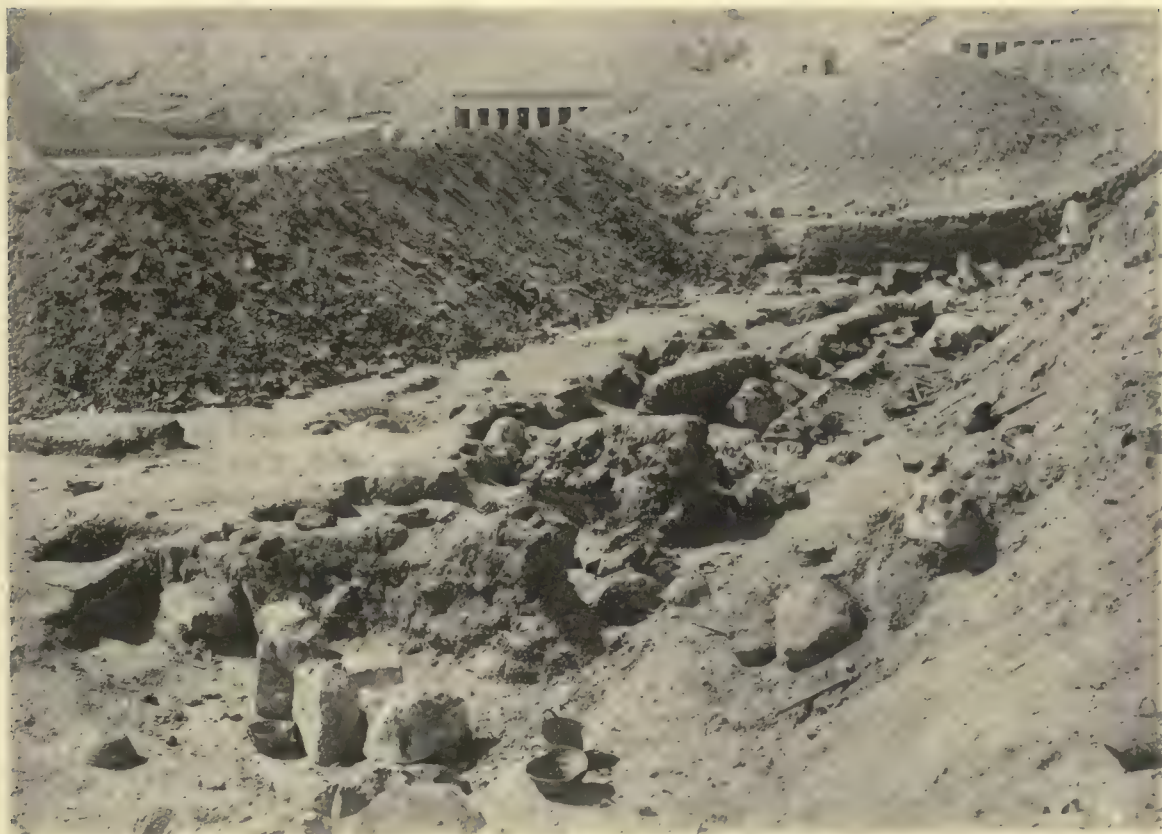
1. FOUNDATIONS OF WALL OF AMENHETEP I AND AAHMES-NEFERT-ARI, AND WORKMEN'S DWELLINGS
